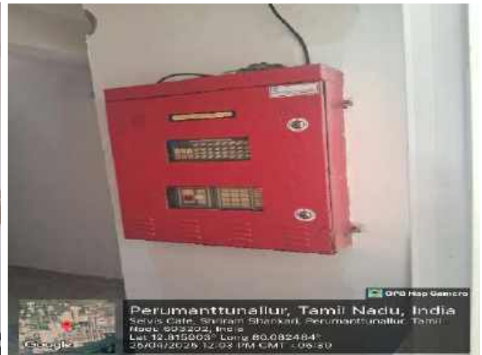
Emergency Fire Alarm System
